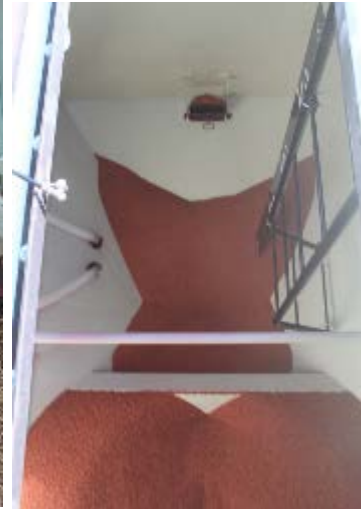
No build up or staining
